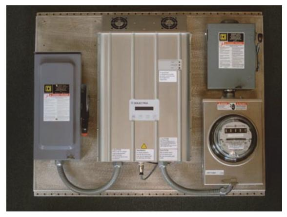
Fig. 7 A typical PVI 1800 or PVI 2500 installation with AC and DC disconnects. (AC disconnect is on the right, DC disconnect on the left. PVI 2500 shown.
